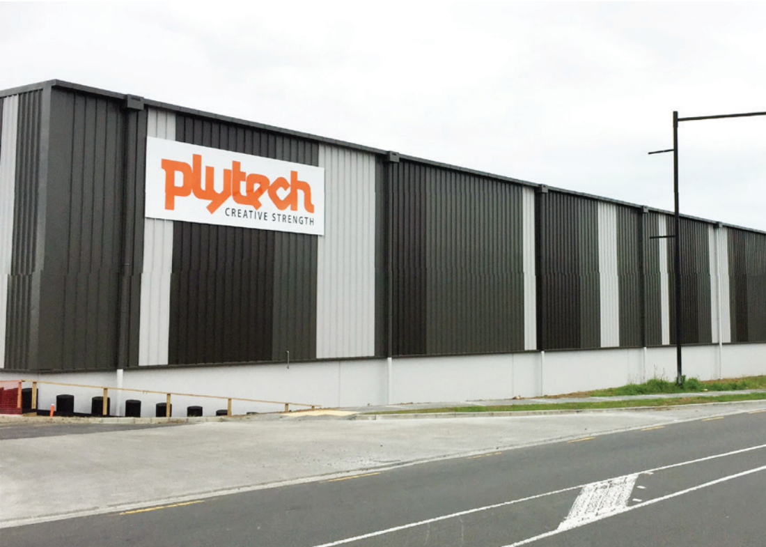
Steel & Tube Roofing Auckland has recently completed a number of large commercial projects in Highbrook, including the cladding and roofing of this Plytech building.
